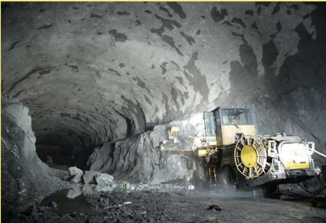
*Excavation of the Bekkelaget sewage treatment plant by drilling and blasting.*
