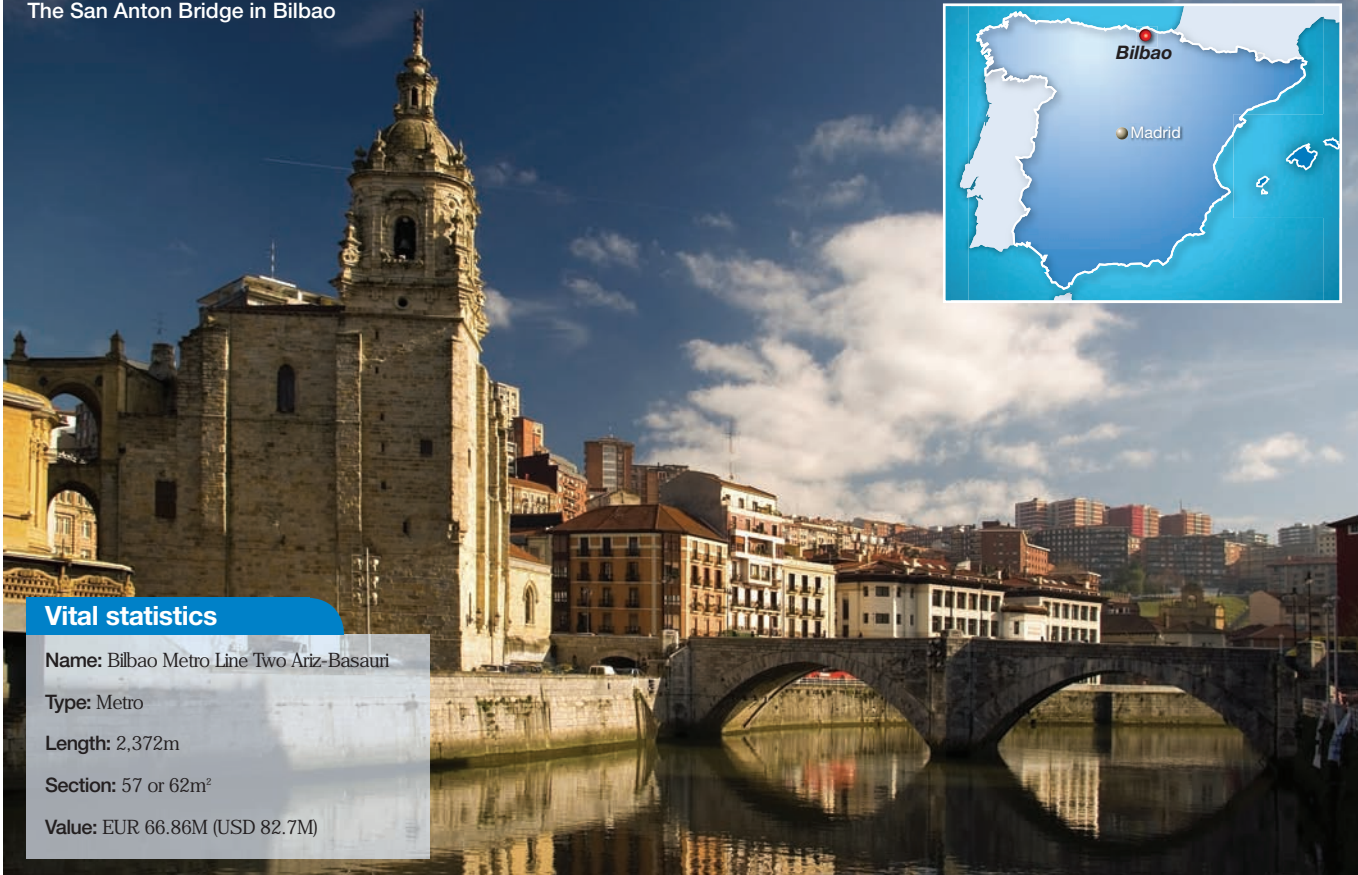
The San Anton Bridge in Bilbao
